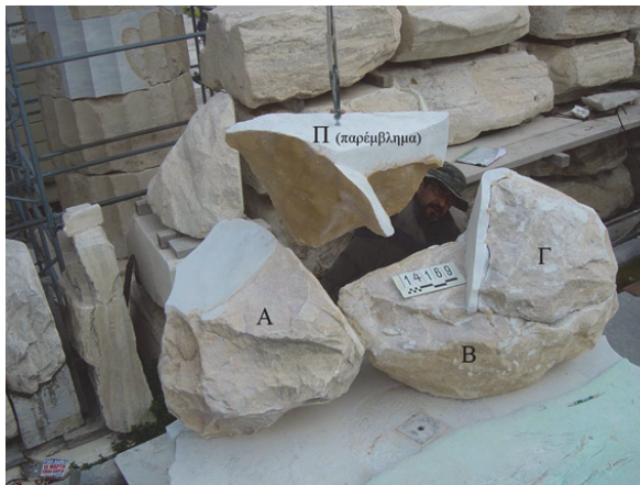
Figure 1: Joining together the ancient fragments A, B, Γ, with the new insert Π to keep them in the right position within the member's volume using cement mortar (left). The joining of this group and the main block of a new marble with "montage" reinforcement bars is presented in the right photo. In the foreground view the opposite fractured surface and the points, where reinforcing bars will be inserted during the next step of intervention, are presented. (Author's note: All pictures in this paper are from the archive of YSMA).
