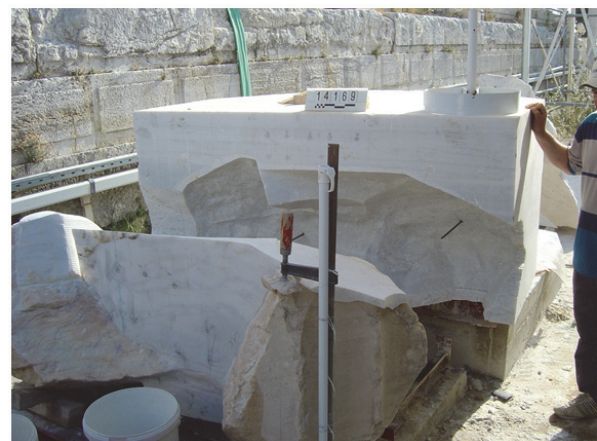
Figure 1: Joining together the ancient fragments A, B, Γ, with the new insert Π to keep them in the right position within the member's volume using cement mortar (left). The joining of this group and the main block of a new marble with "montage" reinforcement bars is presented in the right photo. In the foreground view the opposite fractured surface and the points, where reinforcing bars will be inserted during the next step of intervention, are presented. (Author's note: All pictures in this paper are from the archive of YSMA).
