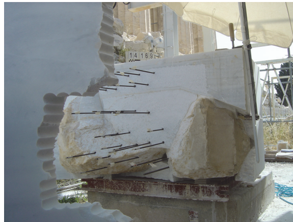
Figure 2: The aforementioned complex is joined to a new supplement along the height of the drum (depicted in the foreground on the left).
