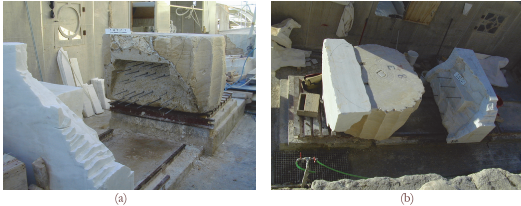
Figure 12: (a) Joining the first supplement. (b) Joining the second supplement. On the left the first -raw- supplement is already joined.
